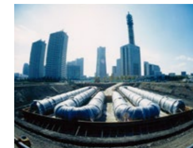
State at the time of installation
