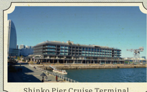
Shinko Pier Cruise Terminal
