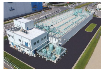
Minami-Honmoku Block #5 wastewater treatment facility
