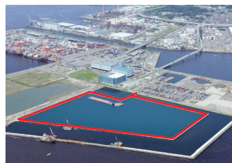
Minami-Honmoku Block #5 Final Disposal Site
