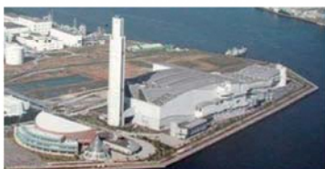
▲Tsurumi Incineration Plant
